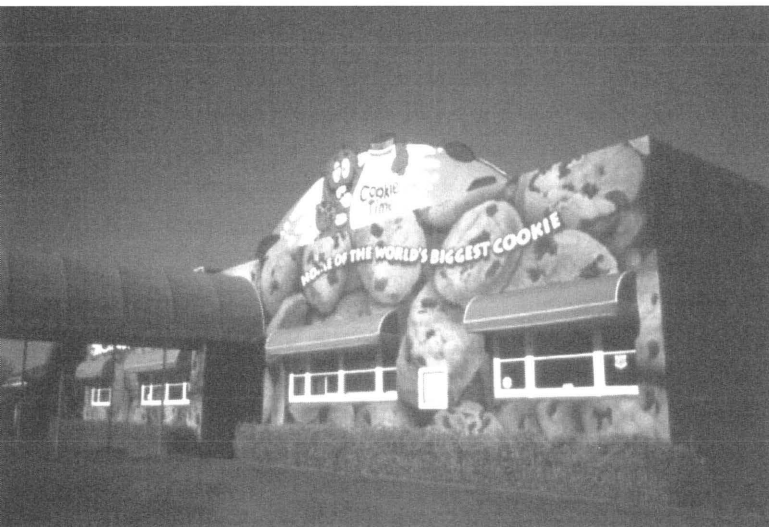
FIGURE 30 Cookie Time manufacturing plant, Christchurch, New Zealand 1999.
