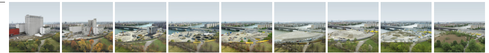
Figure 4.5.2 15.04.2010 / 29.09.2010 / 23.08.2011 / 27.09.2011 / 25.04.2012 / 05.12.2012 / 21.07.2014 / 19.11.2015 / 30.05.2016 Image selection according to traceability of architectural change with assembly of seasons
